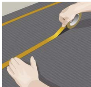
Lay strips of double sided tape to the floor
