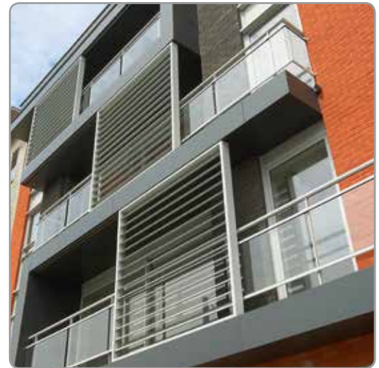
Loggia®, apartments, Kortrijk (BE)
