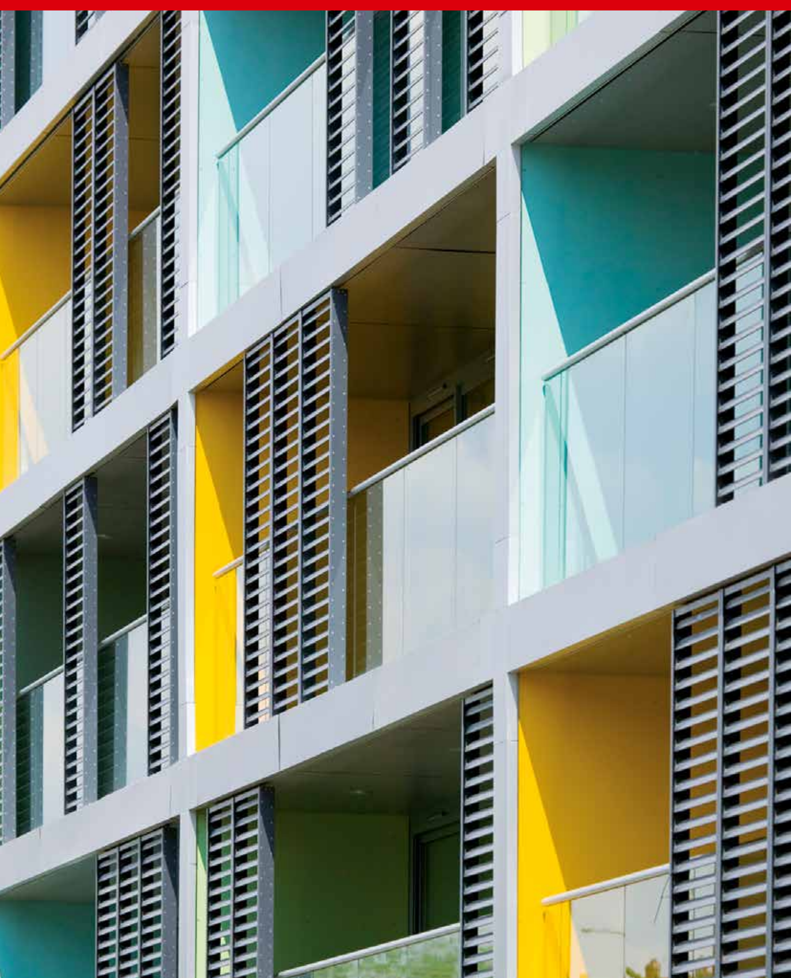
Candy Wharf, Copperfield Road, London (UK)
