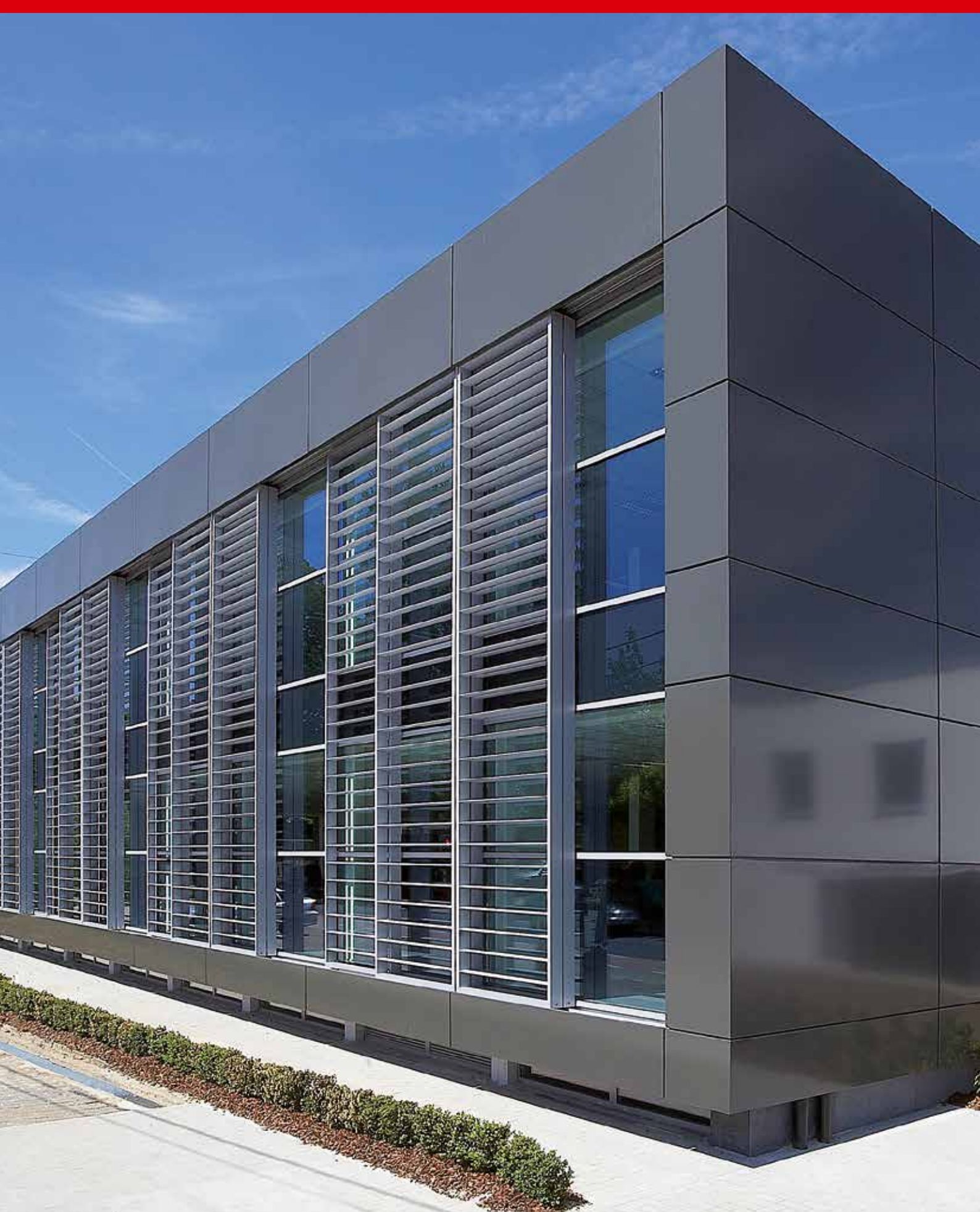
Loggia® 130 with Icarus® 125, TMWV Offices, Asse (BE)
