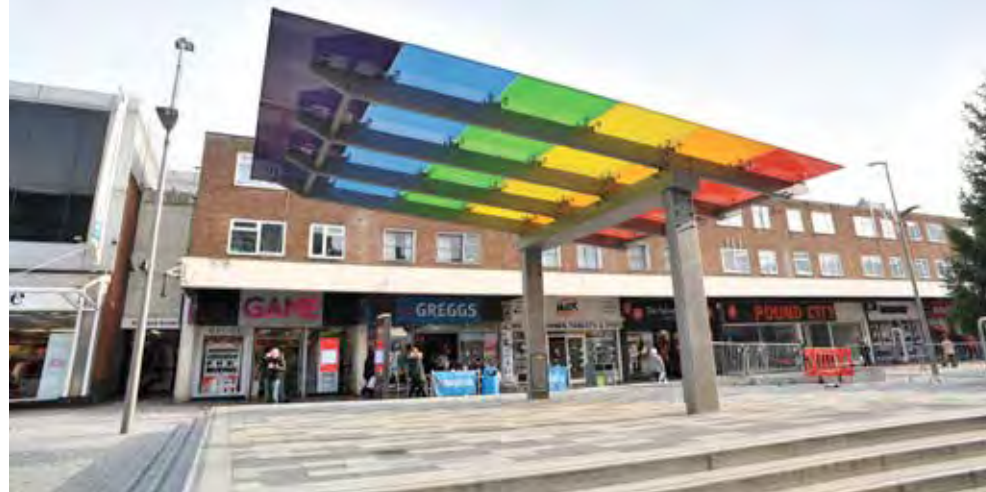
Marlowes Shopping Precinct, Hemel Hempstead
