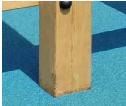
Root fixed timber posts.
