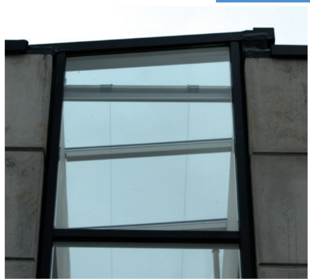
Em-Glaze horizontal to vertical glazing detail
