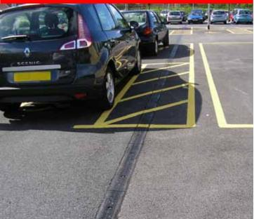
The 750 bed Morriston Hospital, Swansea NHS Trust, car park is drained by 850 metres of RECYFIX® STANDARD 100 channels fitted with HEELSAFE ductile iron gratings. The channels are moulded from the company's tough recycled polyethylene-polypropylene (PE-PP) which is resistant to UV and road salt.
