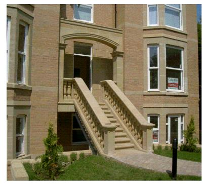
Cast stone balustrade, steps and ashlar were purpose made to the architect's design to create this imposing entrance feature.
