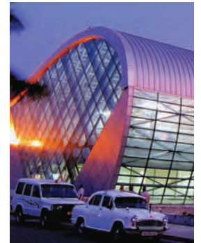
Mumbai Airport, India
