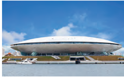
Shanghai Expo Performance Centre, China
