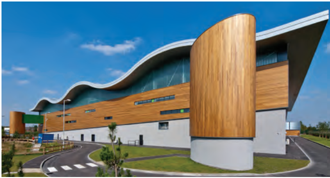
Energy From Waste, Gilmoor
