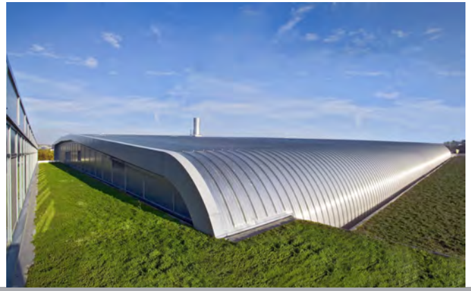
Lough Road, Water Treatment Works,
