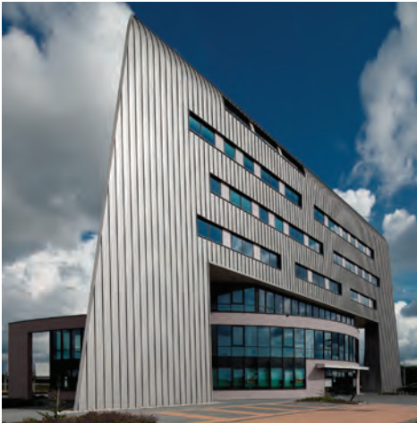
Office Building, The Netherlands
