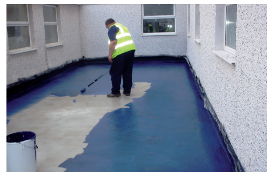
Application of Newton 902 Primer to prevent outgassing from the new concrete
