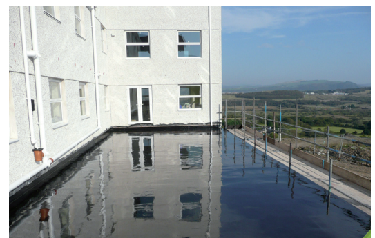
Application of Newton 201 RubberFlex liquid waterproofing membrane
