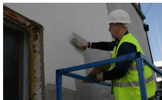
Mineral based breathable top coat applied to Diathonite insulating plaster
