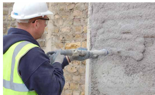
Diathonite insulating plaster professionally sprayed by trained applicators
