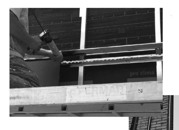
Fixing with chemical anchoring on profiles.
