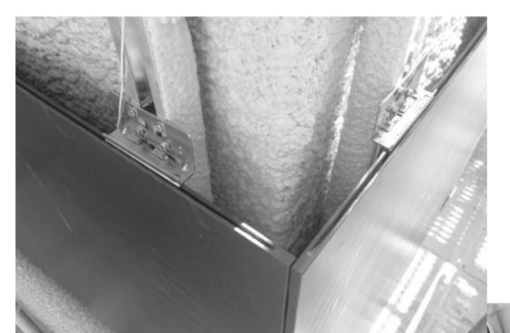
Dekton® has the certification for ventilated façades according to ETA 14/0413 and BBA 16/5346 for 12mm and 20mm thicknesses, although it can be used for other non-certified thicknesses.
