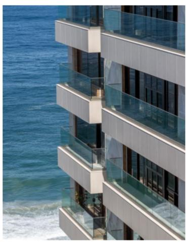
Di Filippo Arquitectura chose Dekton® by Cosentino for the façade for various reasons: it represented just 50% of the permitted load for the material, it can be manufactured in large format, bespoke slabs (3.2 m  $\times$  1.44 m), the precision cutting of pieces, its optimal performance against sand and saltwater erosion from the beach, and its other exceptional qualities such as its high resistance to ultraviolet rays, its colour stability and high resistance to stains.
