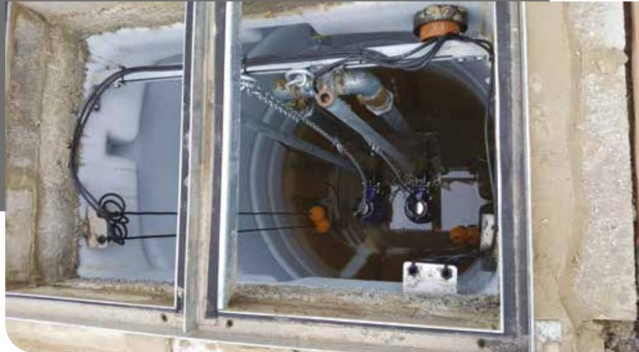
Our range comes in both single and twin pump configurations and in a variety of tank sizes. There is also a wide range of pumps/control options available to suit your precise requirements. With the SumpFlo and DrainFlo ranges, Wykamol can assist you with all your basement pumped drainage requirements.
