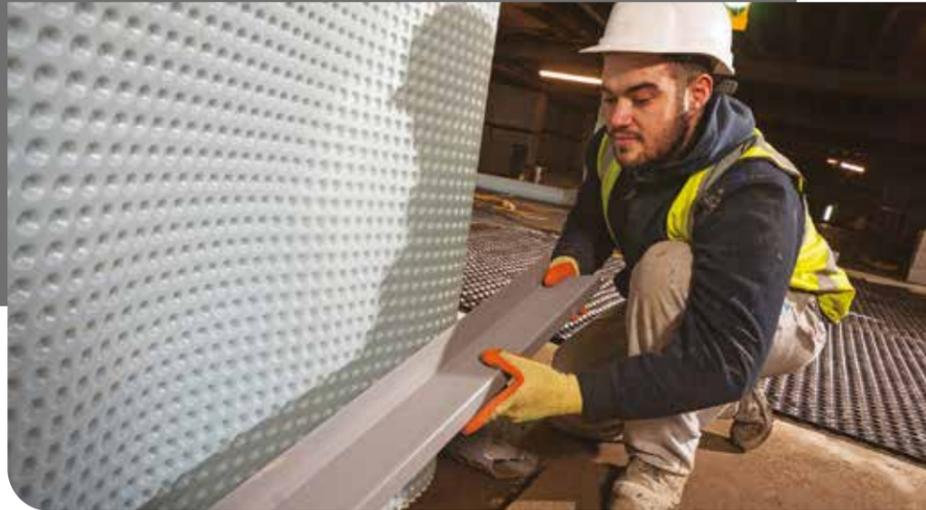
As part of the Wykamol cavity drain membrane system, channels are a crucial part of the overall system, and are laid at wall floor junctions to remove any water entering the structure.
