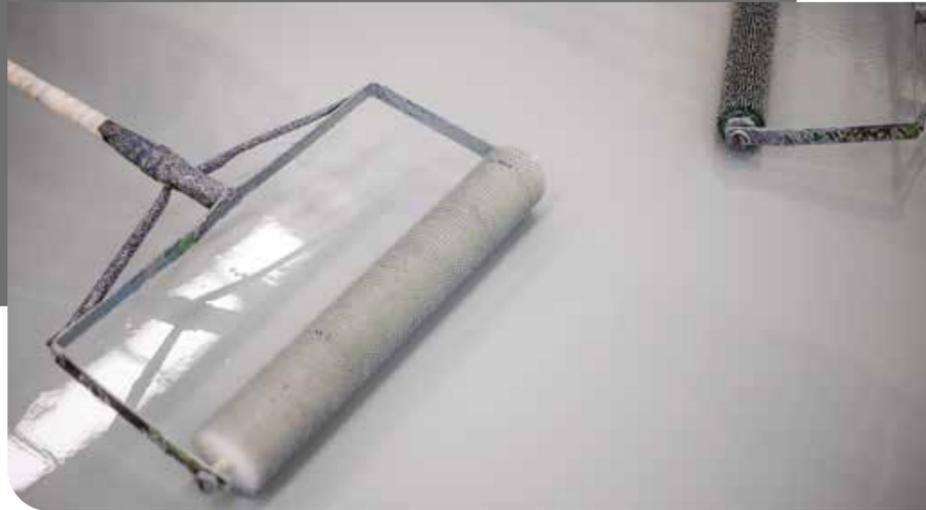
EP40 Floor Coating System is a water-based, easy to apply system which consists of the EP40 Epoxy Floor Primer and the EP40 Epoxy Finish Coat in grey or clear.
