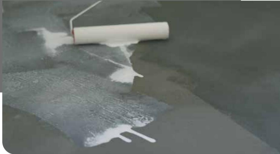
Wykamol Anti-Lime sealer is applied to concrete and cures to form a water repellent surface which is resistant to lime efflorescence.
