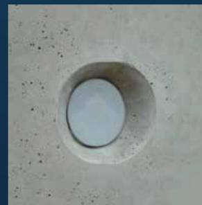
The Sealing Plug is designed to offer a more effective, quick and secure sealing solution than mastic or a length of water bar – both of which can be dislodged during the concrete pour.
