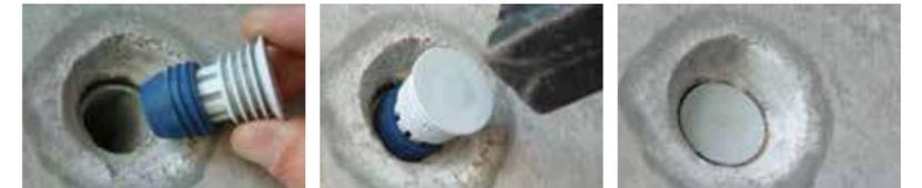
Position the Sealing Plug in the formwork spacer
