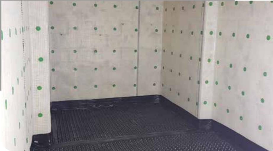
Wykamol **CM Plaster Plugs** and **CM Brick plugs** are of a high quality and can be used in a range of applications and on multiple substrate types. The tailor made Thermoplastic Elastomer seal ensures application of the membrane is water tight, if a normal fixing cannot be made then our **COB plugs** are ideal.
