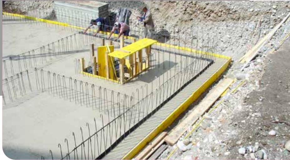
**Cemflex VB Plate Steel Waterbar** is a galvanised steel plate encapsulated in a special patented coating that reacts only with the water within the concrete to provide a watertight joint.
