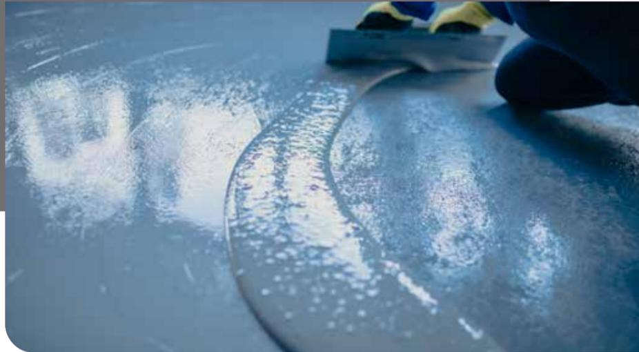
A solvent free, two-part epoxy resin coating primarily for use on screeded or concrete floors subject to rising damp or containing residual construction moisture.
