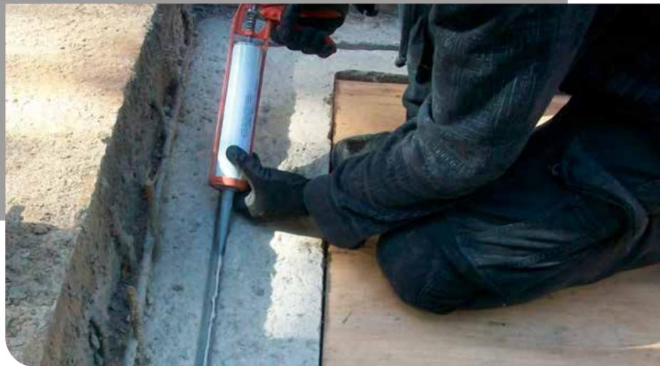
Hydrophilic Waterstop and Adhesive, a grey, elastomeric, water-swellaible paste which is applied like a sealant.
