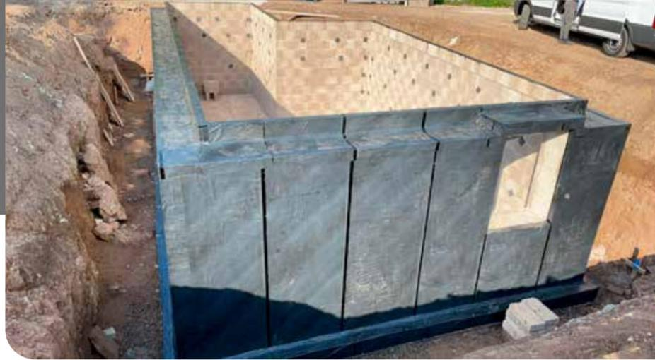
The high-density polyethylene film gives to the membrane characteristics of dimensional stability and ensures a uniform reaction to elongation stresses in a longitudinal and transversal direction.
