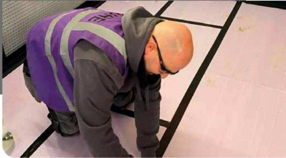
Wykamol HIGH LOAD Thermal spacer has been specifically developed to assist in the installation of internal waterproofing systems for basement structures.
