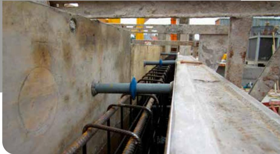
The Sealing UFO is designed to offer a more effective, quick and secure sealing solution than mastic or a length of water bar – both of which can be dislodged during the concrete pour.
