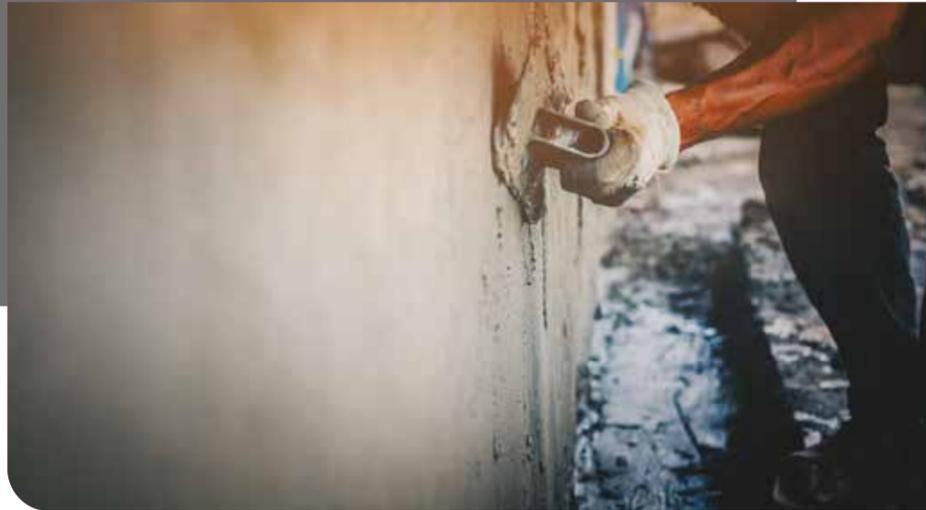
Universal Mortar is a single component, thixotropic, fibre reinforced, polymer modified cementitious mortar.
