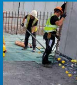
Wykamol Bentonite is a high performance sodium bentonite system.
