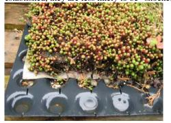
The build-up is the same as with the component green roof, each tray holding the Pro-drain 20P drainage sheeting, geotextile filter layer, approximately 70mm of aggregate based substrate and a sedum blanket.
