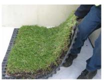
Installation couldn't be simpler. Just protect the waterproofing, lay the bottom layer of geotextile filter fabric and place the module into position on top.
