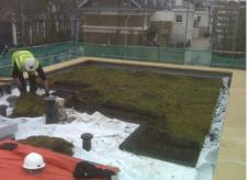
Each module is an established instant sedum roof system in itself, so when all trays are installed, the roof is finished. This cuts down on mess around site and the amount of space required to install the roof. Also, because these plants are fully established, they are less likely to be "shocked" once installed onto the roof and more likely to thrive quickly.
