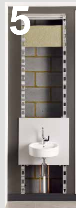
05 Once all the units are in position, connect the plumbing and services.
