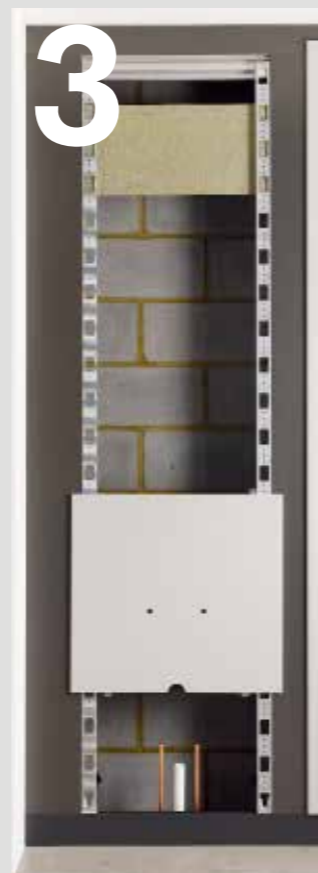
03 Drill or cut out for sanitaryware.
