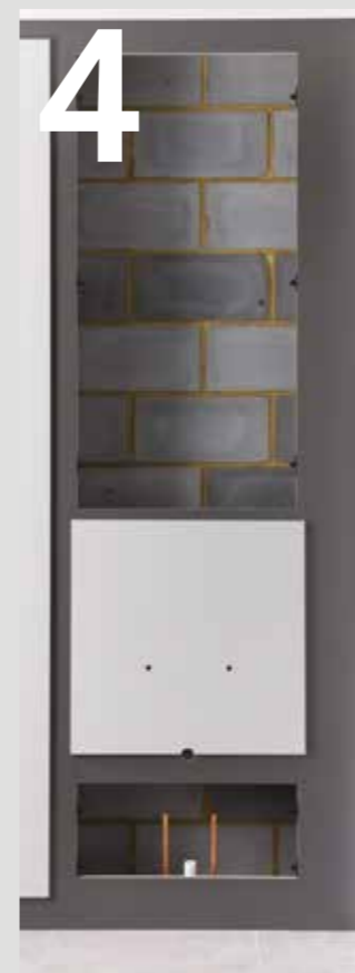
04 Drill or cut out for sanitaryware.
