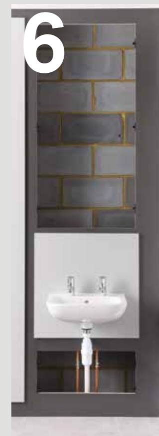
06 Once all the units are in position, connect the plumbing and services.
