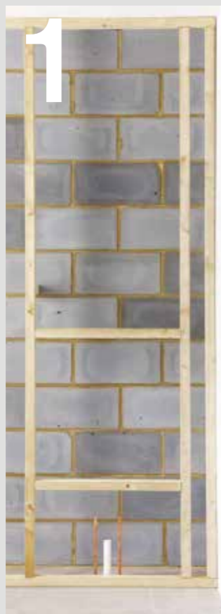
01 Install timber-frame (supplied by others).
