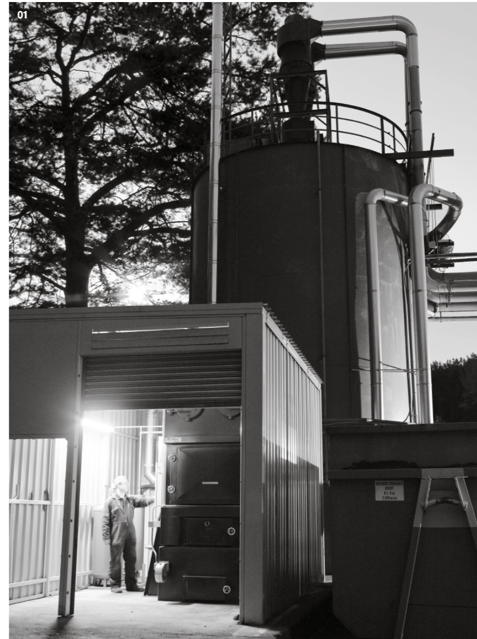
01-03 Waste management Biomass burner turns smaller production waste into factory heating
