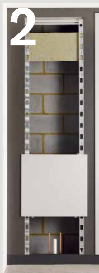
02 Click-fix the first IPS unit onto the frame and slide into position. Attach a vertical flashgap to the frame, on either side of the unit, screw-fixing to the frame from the face. Fix tie back to the wall. Repeat until all units are in place.
