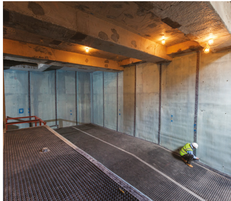
Platon P8 cavity drain membrane shown installed to walls
