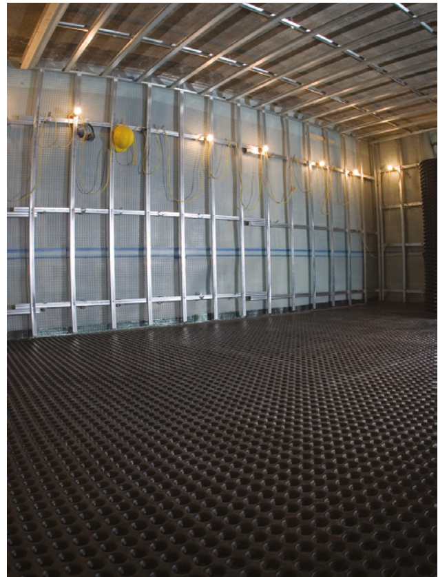
A fully sealed Type C system showing cavity drain membranes installed to walls and floor
