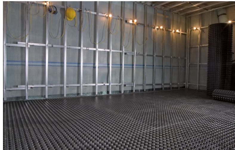
Platon P20 membrane shown installed to floor
