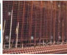
Installed in cavity walls, DELTA®-MS 20 provides reliable drainage.
