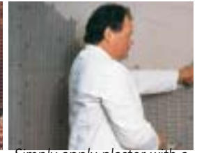
Simply apply plaster with a trowel.
