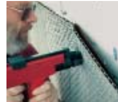
A typical way of installation is to attach the dimpled sheet with a gas or nail gun.
