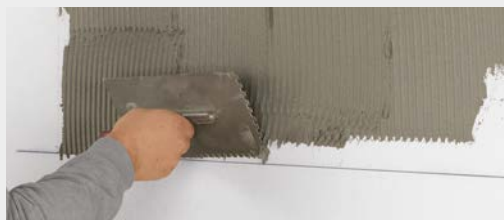
Apply the ready-mixed mortar
