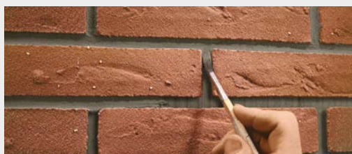
Smooth out the joints - Done!
