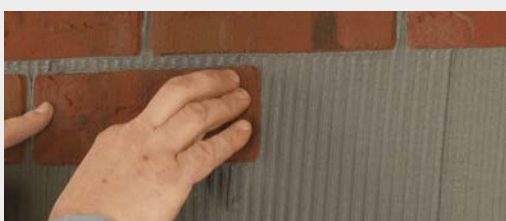
Apply the StoCleyer B slips
