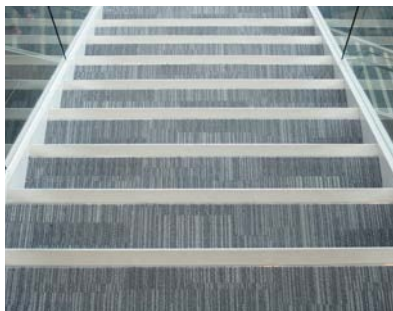
Good Visual Contrast Installed with Gradus Stair Nosings picture 1
