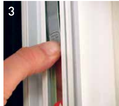
3) Once the safety catch is released the window can be completely rotated.
