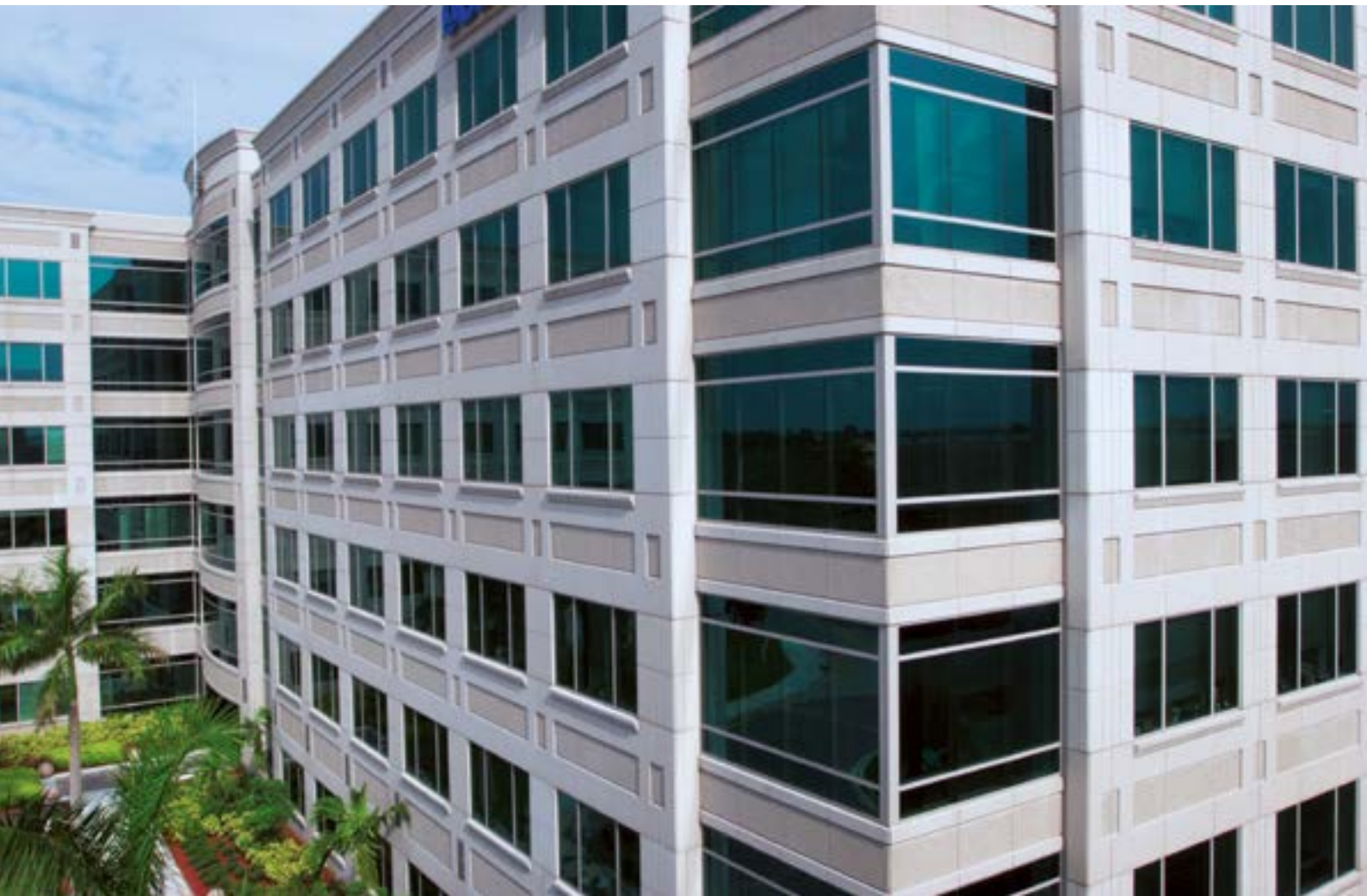
• BellSouth building, Fort Lauderdale, USA
