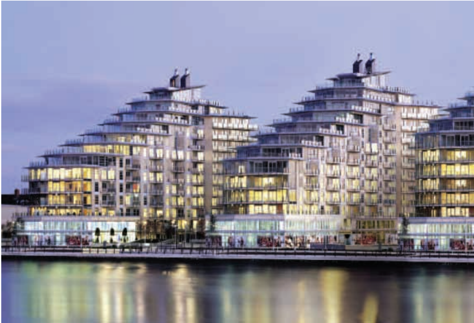
ABOVE: Battersea Reach LONDON
