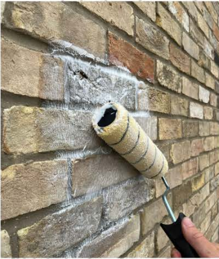
5.1.2 Roll applied Passivhaus Brick Seal
