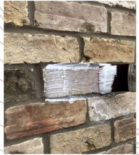
5.1.4 Brush applied Passivhaus Brick Seal
