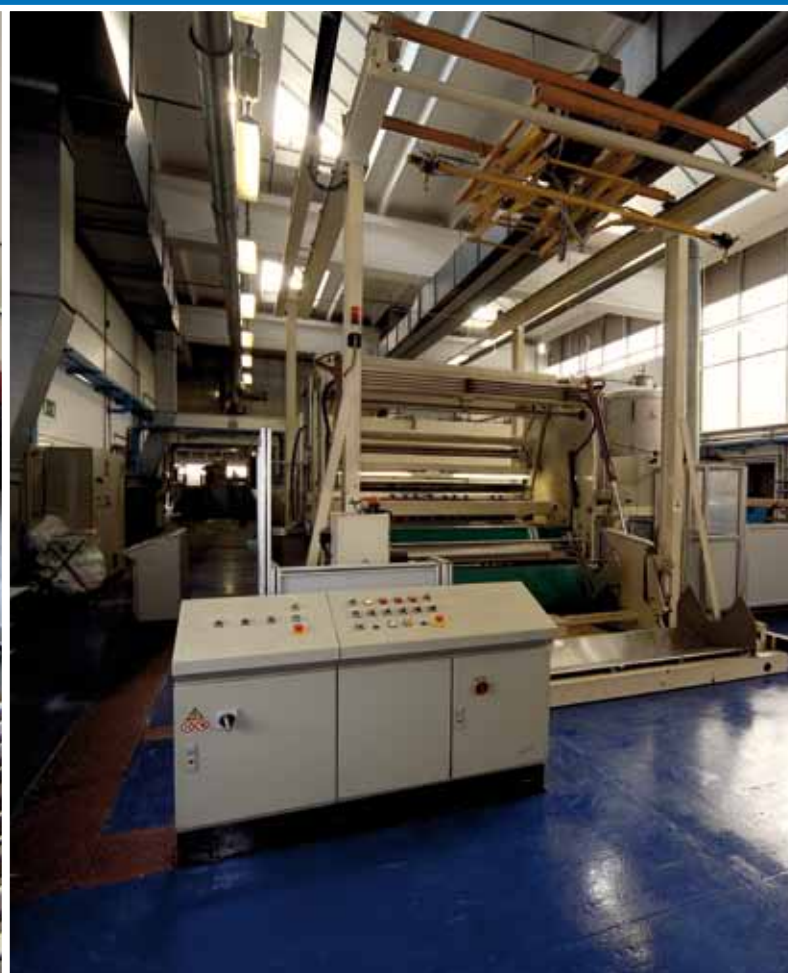
Sisma storage depot - Bollate (Milan) - Italy Products used: MAPEFLOOR SYSTEM 32
