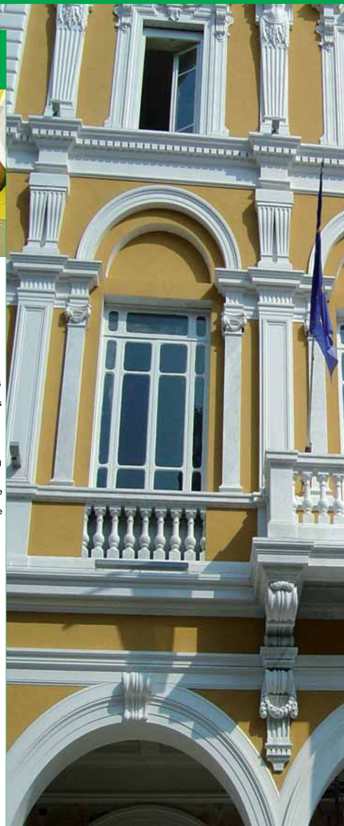
Palazzo Zaccagna - Carrara - Italy Protection and decoration of the façade with: Elastocolor Paint, Silancolor Tonachino
