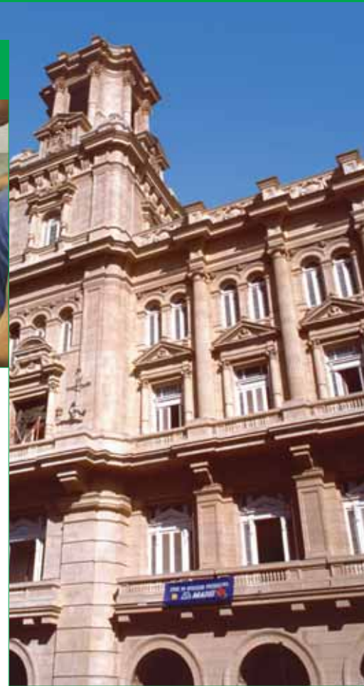
Asturiano Centre Building - Havana - Cuba Reparation and protection of the building façades with: MAPEGROUT THIXOTROPIC , MAPEFER , MAPE-ANTIQUÉ FC , MAPE-ANTIQUÉ MC , MAPE-ANTIQUÉ LC , SILEXCOLOR PAINT
