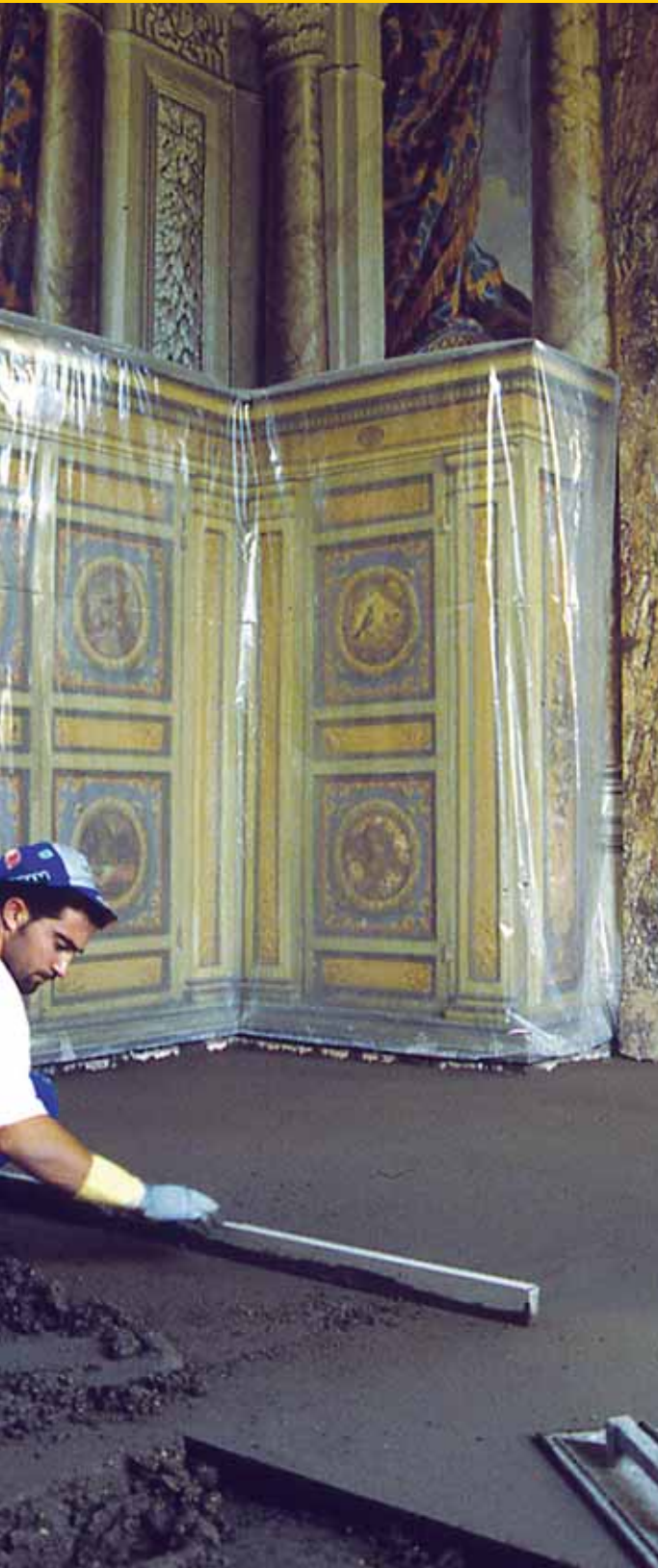
SISTINE HALLS - Vatican City Products used: GRANIRAPID, ULTRACOLOR and MAPEFLEX PU21 were used to install porcelain tiles over MAPECEM screeds
