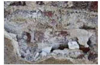
Typical damage through salt efflorescence.
