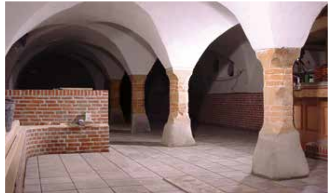
Typical damage through salt efflorescence.
