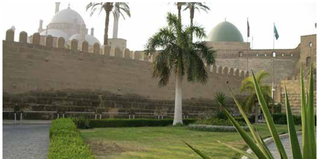
Example of rising damp
