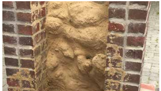
Curtain Injection (rear view)
