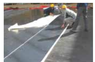
Waterproofing with KÖSTER KSK
