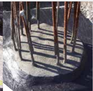
Connection of the area waterproofing (KÖSTER Deuxan 2C) to the pile head waterproofing.
