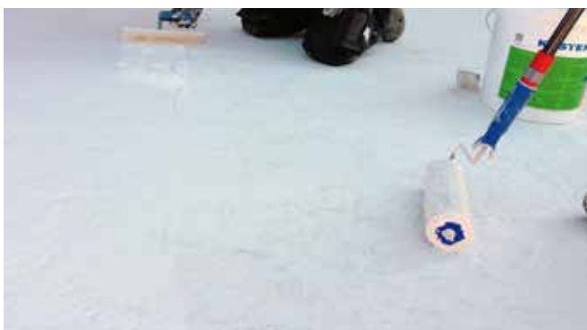
Application of the second layer of KÖSTER 21
