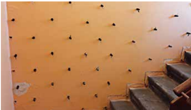
Injection into Concrete
