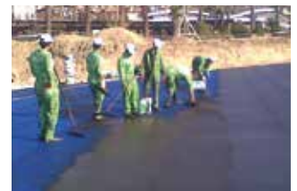
Waterproofing with KÖSTER Deuxan 2C
