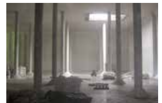
Positive waterproofing of a tank with KÖSTER NB 1 Grey
