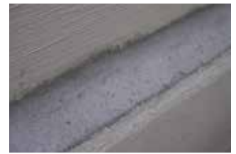
Round fillet made of KÖSTER WP Repair Mortar
