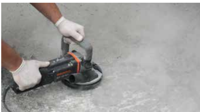
Substrate preparation
