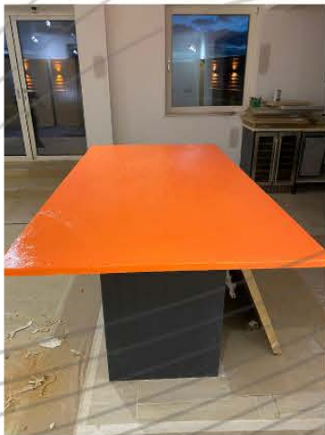
5.1.5 Phuck off kitchen island install
