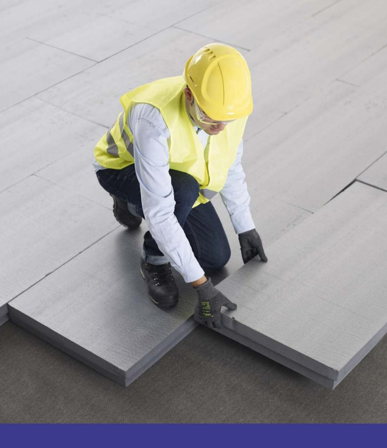
Ravatherm XPS X has been created specifically for inverted roofs – a form of flat roof where the thermal insulation is placed above the waterproof membrane. The added benefit of this type of roofing is that the membrane is also protected from expansion and contraction caused by changes in the weather and temperature. The inverted roof system is ideally suited to flat roofs of heavyweight construction, and offers a durable, attractive roof finish for roofs where maintenance traffic is expected.
