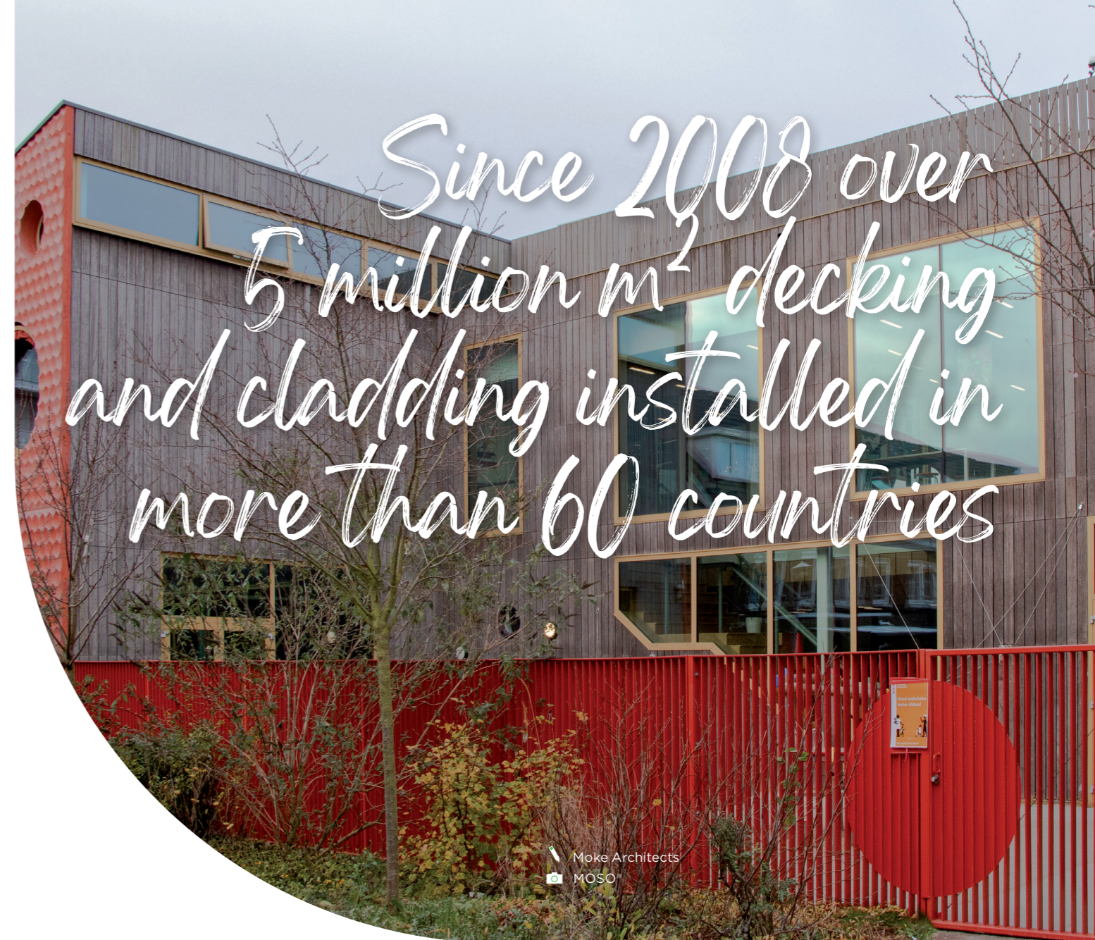
Public Elementary School "IKC" Photo taken 5 years after installation - (320 m²) Amsterdam, The Netherlands
