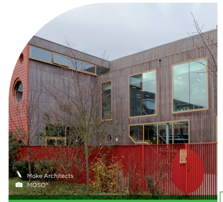
Public Elementary School "IKC" (320 m²) Amsterdam, The Netherlands
