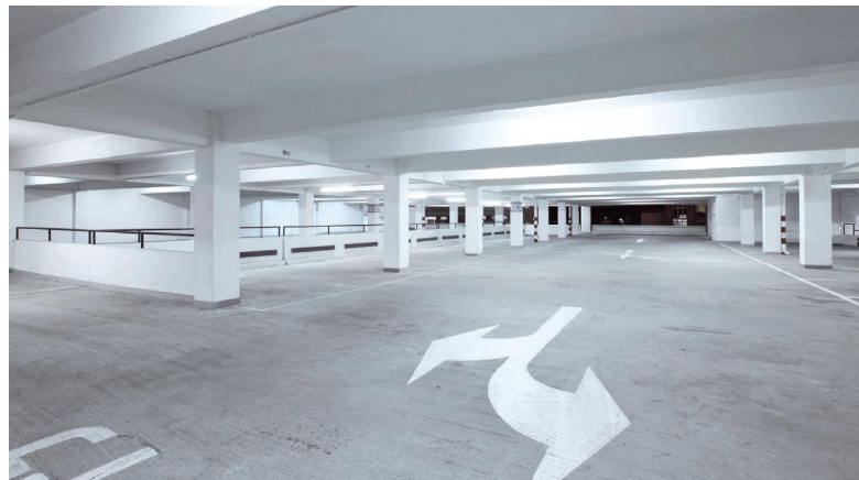
UNDERGROUND CAR PARKS
