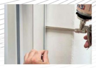
The joints can now be almost completely filled with a suitable insulating material.
