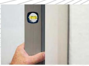
Now align the window and check the joint width again.
