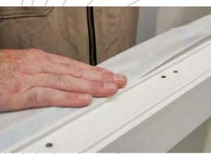
Peel off the narrow liner section from the adhesive and press Intelligent Membranes®- Airtight Fleece Tape well to the window frame. It may be necessary to clean the surface of the window profile before to remove any production film or condensation. Please ensure there is sufficient attachment to the window frame and the window fins respectively.
