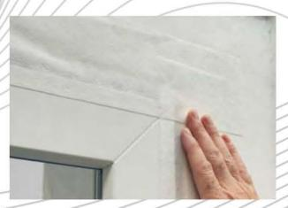
Ensure a minimum adhesion width of  $\geq 15$  mm (5/8") on the surface of the window frame.
