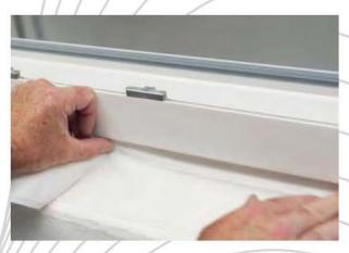
To seal the bottom joint, remove the narrow liner strip and press the tape to the window profile.
