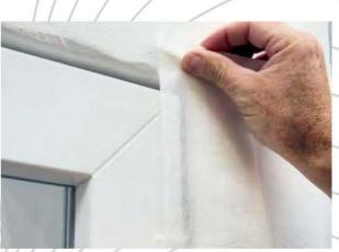
With the moisture-variable Intelligent Membranes®-Airtight Fleece Tape you van seal both the internal and external connection. Alternatively special Intelligent Membranes®- Airtight Fleece Tape for exterior respectively interior applications can be used.
