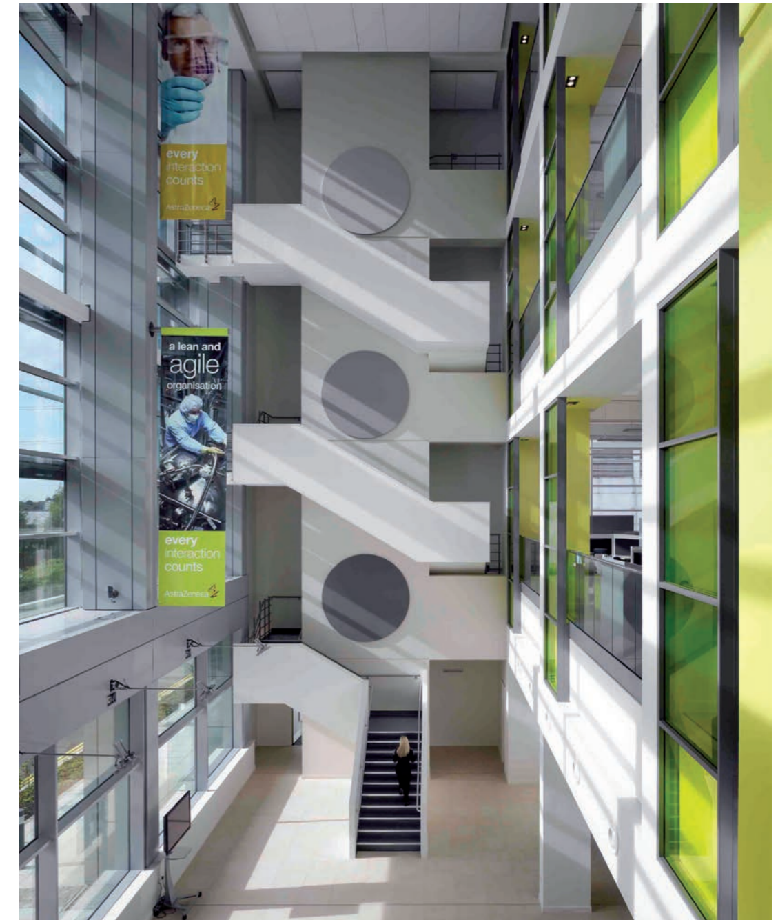
A range of acoustic products have been used in this atrium to reduce reverberation. As well as an acoustic ceiling, the wall discs and the panels below the glass barriers are made of sound absorbing material.
