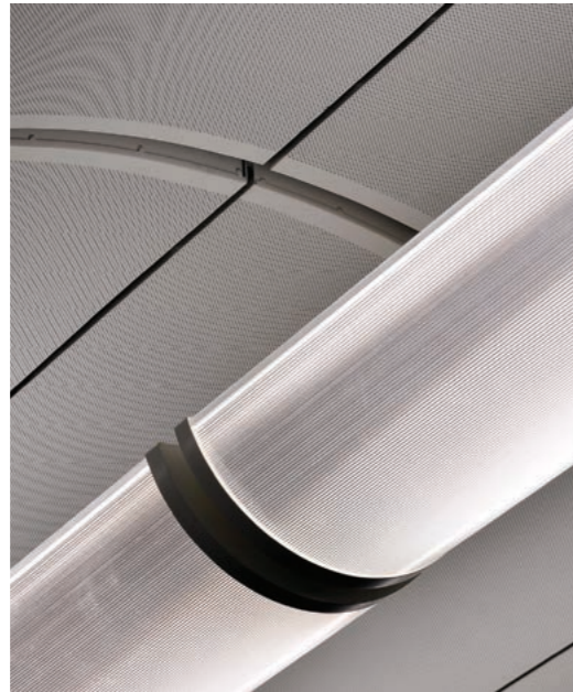
Acoustic waveform panels with integrating lighting detail
