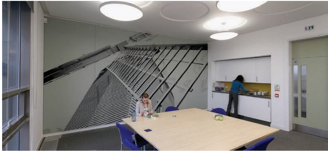
Acoustic wall panels with digitally printed fabric covering.
