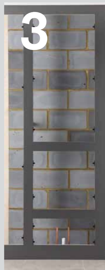
03 Attach fixing clips to the inside edge of the vertical flashgaps, repeat process on back face of panels.
