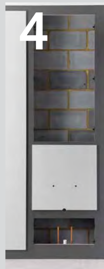
04 Drill or cut out for sanitaryware.
