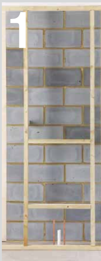
01 Install timber frame (supplied by others).
