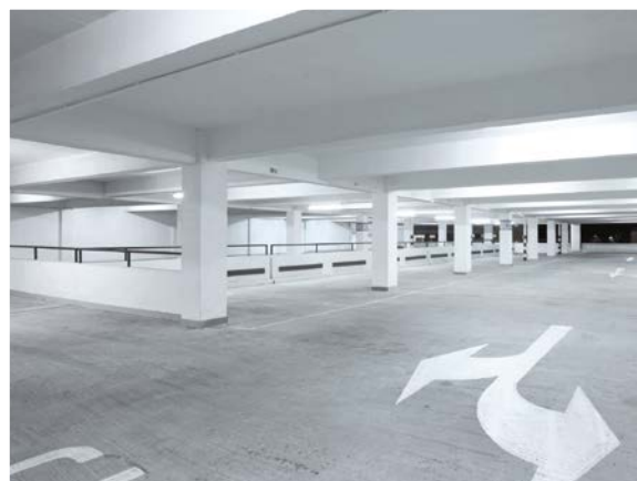
UNDERGROUND CAR PARKS
