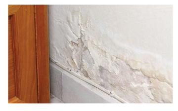
Dampness as a result of hygroscopic salts without any free or capillary moisture, is often referred to as salt damp. Visual evidence of salt damp will be dependent on humidity levels. Hygroscopic salt contamination of the plaster work may sometimes be detected with the aid of an electronic moisture meter even if the surface appears visually dry.
