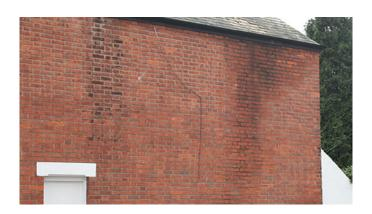
A full understanding of the distribution of dampness in a structure will normally require the use of various moisture measuring techniques. Surveyors should be familiar with the use of such equipment and interpretation of the results produced. It must be recognised that electrical moisture meters will produce only qualitative and comparative readings in masonry. These readings may also be affected by salts.
