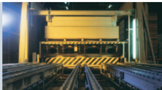
A finished raw panel exits the dryer
