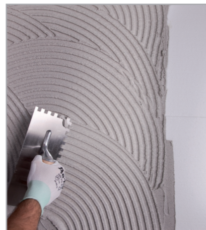
Apply the first coat of the smoothing and levelling layer
