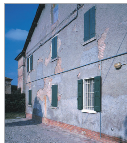
The areas of loose render must be removed before bonding the insulating panel
