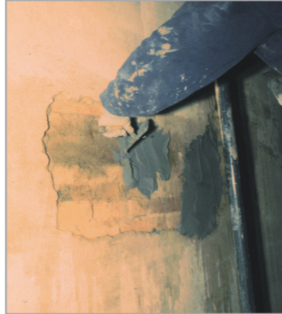
Remove & replace with NIVOPLAN+PLANICRETE
