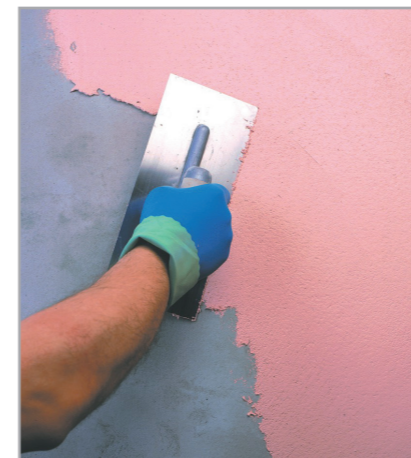
Apply the finishing layer of render
