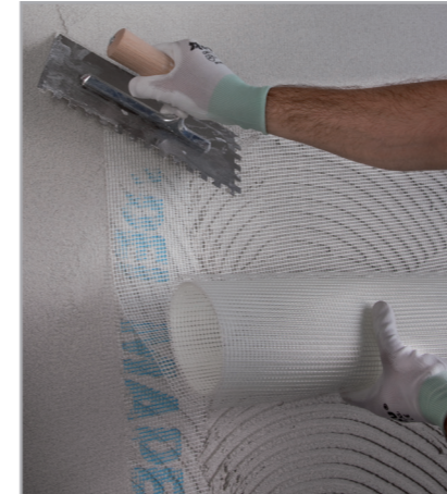
Overlap the edges of the net by at least 10 cm
