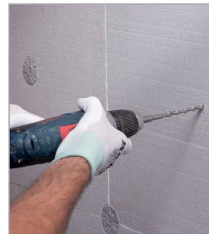
Drill holes for the plugs
