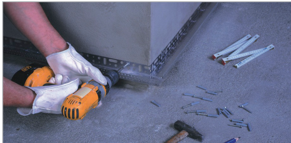
Fasten the support profiles in place using expansion plugs
