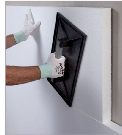
Press down the panel with a float
