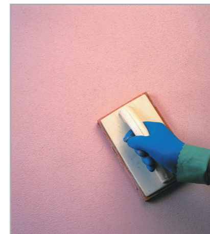
Finish off the surface of the render with a sponge float
