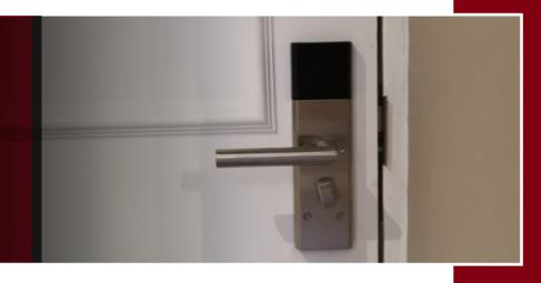
Dialock has been fitted on all guestroom doors, as well as on the main entrance door to the building. The main entrance is controlled by the Dialock WT210 wall reader, a mains operated wall terminal for offline operation. The entire set-up is controlled via the Dialock Hotel software management tool.
