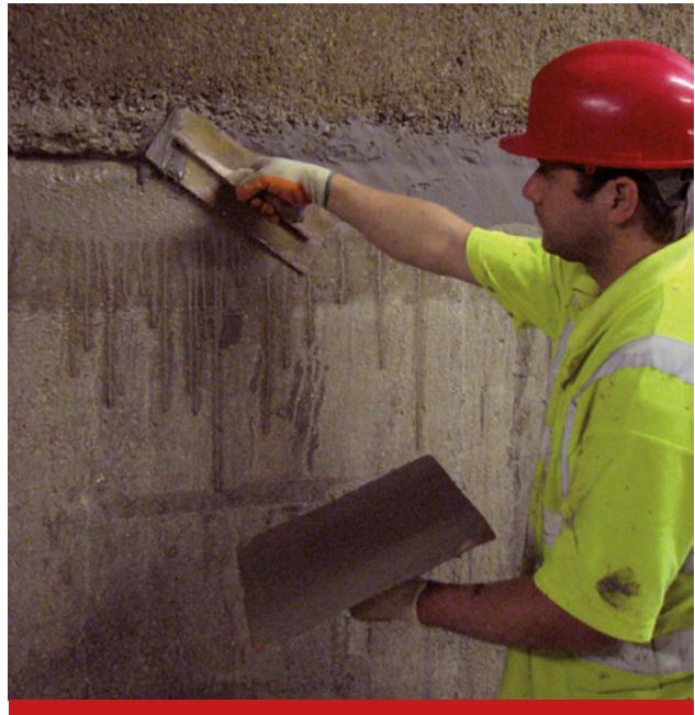
Construction joint repair using Triton Fillet Seal.
